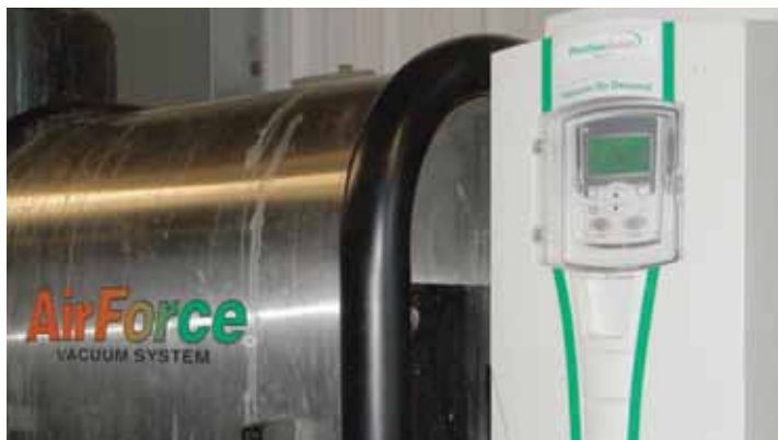
A variable-drive vacuum system and control panels monitor and control milking for each of the 28 cows in the parlor at any given time.
