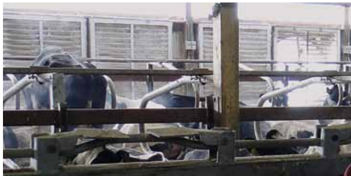
Switching from 108 1.5-hp ventilating fans to 72 1-hp NEMA high-efficiency fans brings substantial energy savings.
