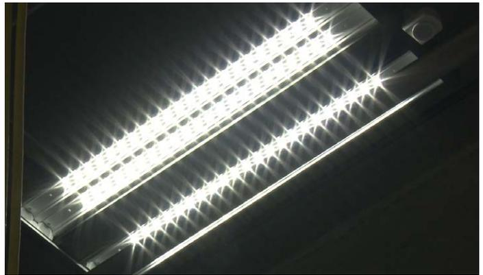
Each LED fixture contains 88 individual LEDs.
