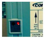
**Both RED lights** indicate water heater and electric heating /cooling are being controlled.
