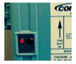
**Right RED light** indicates electric heating/cooling is being controlled.
